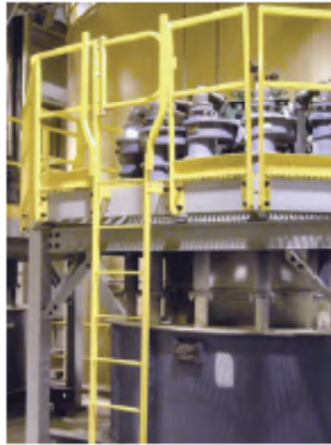
Raised platform with protected guardrail.
